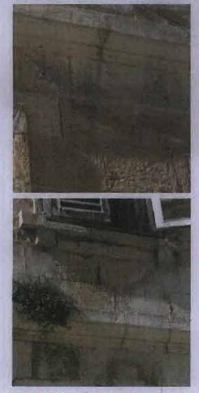
The historic stables - efflorescence and differential erosion.
