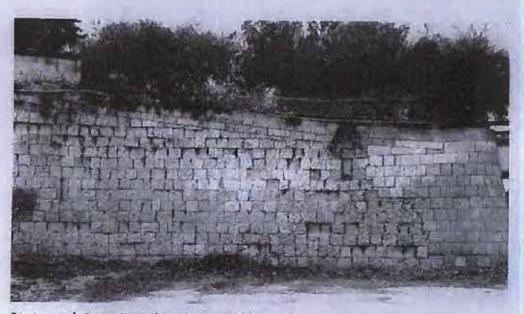
Counterscarp facing south-east showing further surface erosion.
