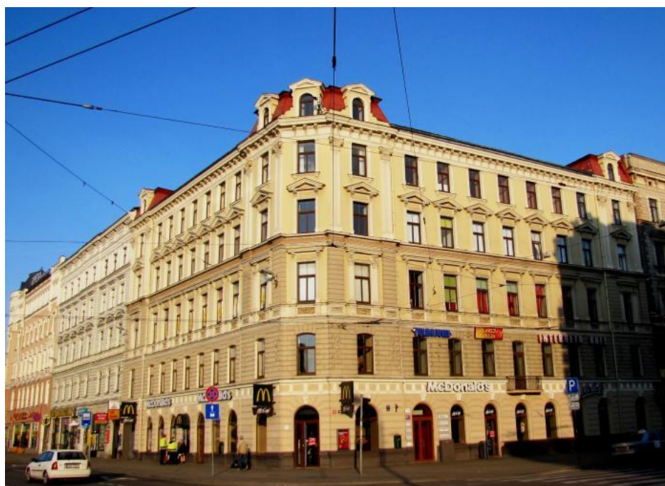
Commercial & office building – Merkela Street, Riga, Latvia
