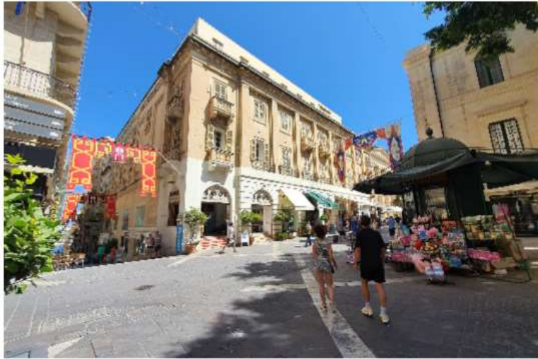
pic6 front facade from corner
