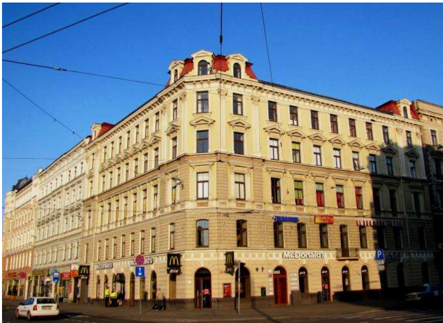
Commercial & office building – Merkela Street, Riga, Latvia
